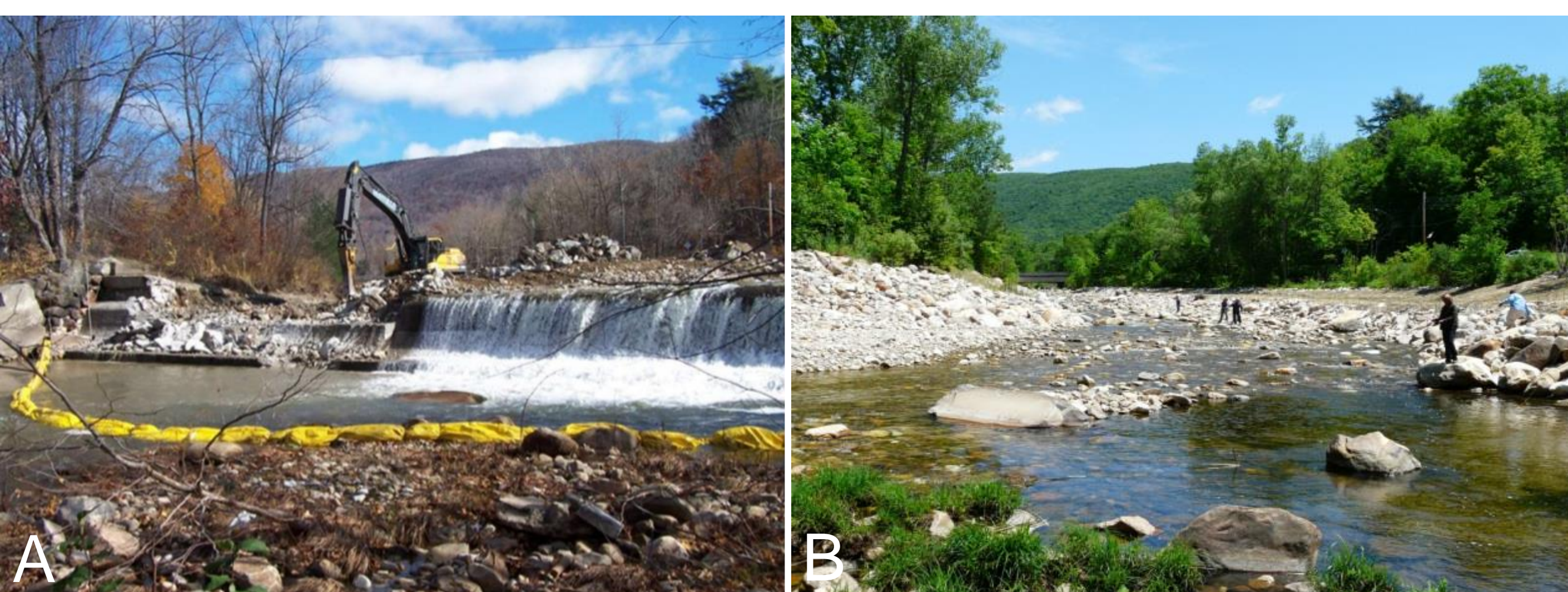
Figure 1. (A) The sediment-filled impoundment of the Briggsville Dam on the Hoosic River in Clarksburg, MA, during removal in 2011. Photo from Buzzards Bay Coalition. (B) Riprap-stabilized banks at the former dam site.
